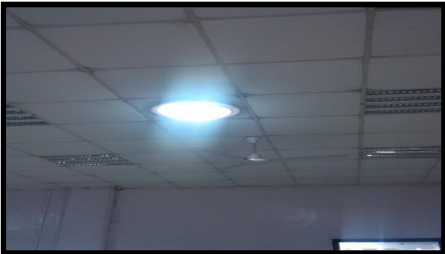
3. DAYLIGHT LIGHT PIPE SYSTEM IN SUB-ASSLY & CE AREA.
